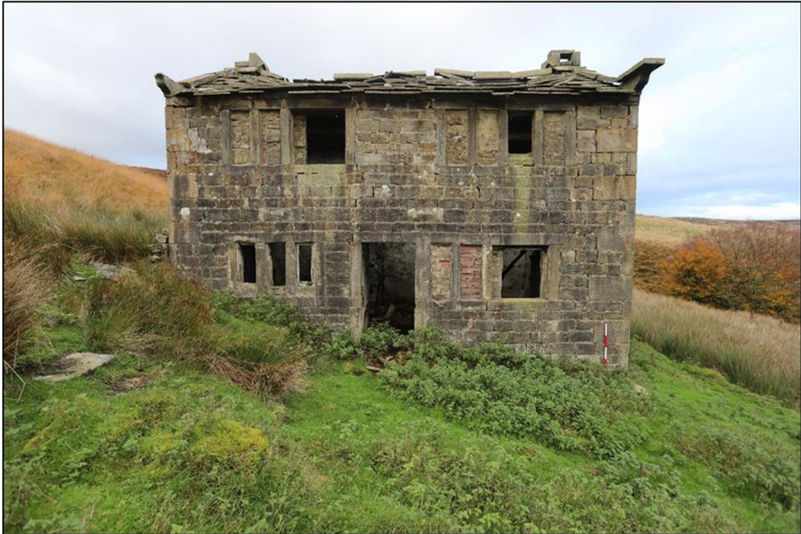
Photo 16: Location of the former Cascade Farmstead (MWY10270), west building, looking north
