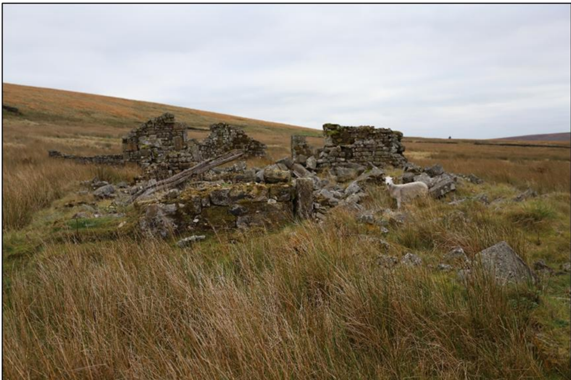
Photo 15: Location of the former Upper Good Greave (MWY3434) looking southeast
