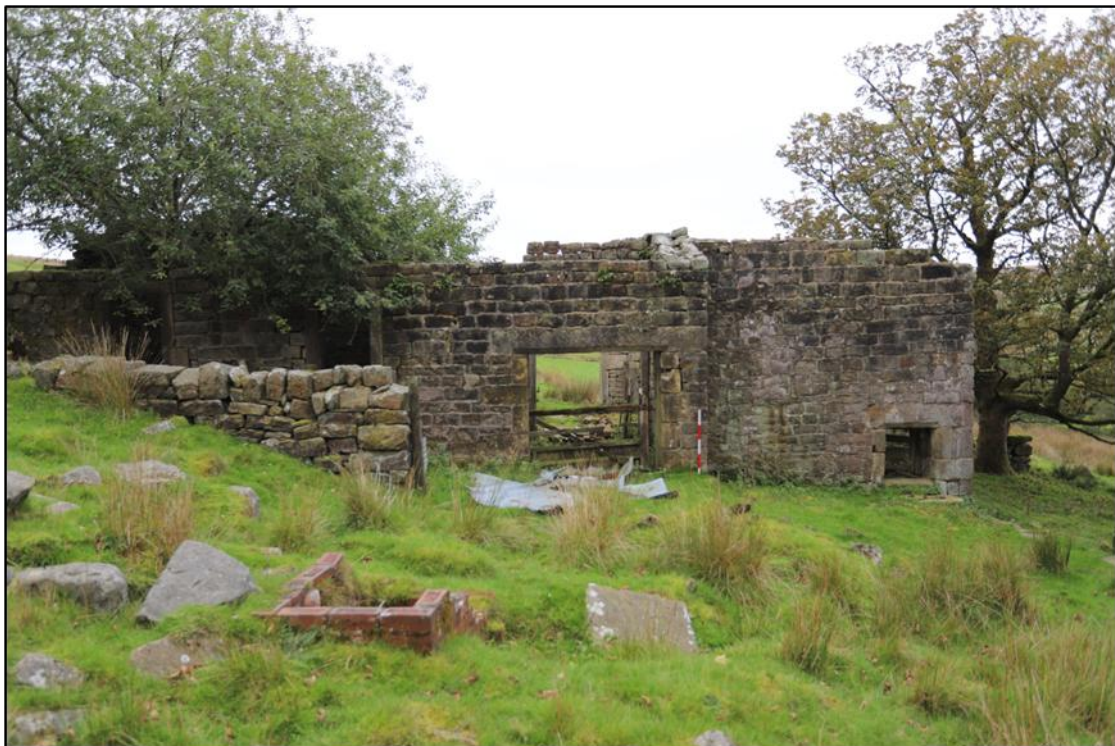
Photo 8: Derelict building illustrated as "Lower Lathe" on the 1851 OS Map looking south
