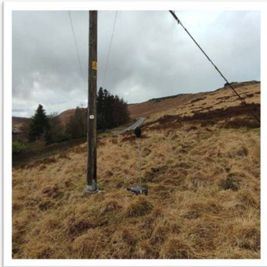
NML01: Looking West
